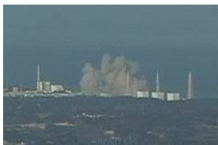
Leakage from the reactor due to effect of Tsunami
