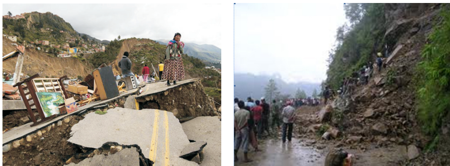
Fig. 30.6 Soil erosion and landslides from mountain heights not only block traffic but also damage habitation
