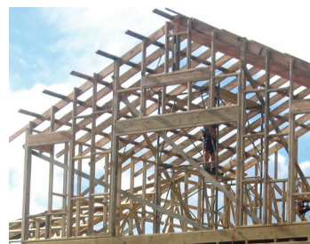
A Building under Construction
